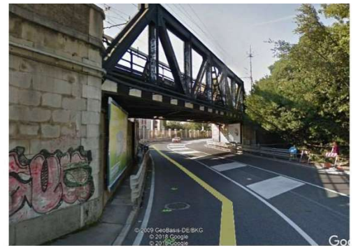
Cavalcavia ferroviario Railway overpass
